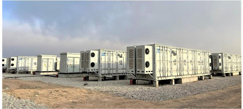
solve the volatility and discontinuity of new energy power generation, ensuring the safe and stable operation of the power system.
